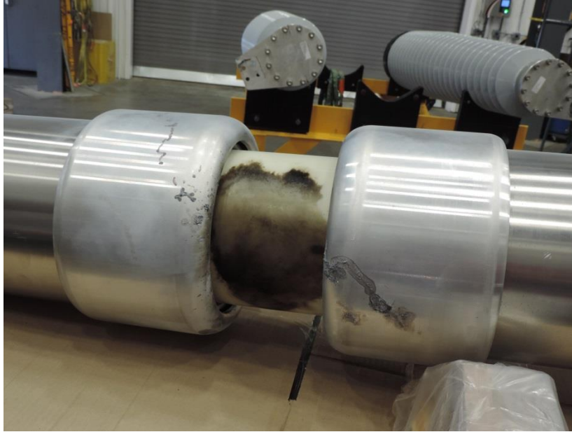
Figure 5: Flash To Ground and Across Insulator Gap
